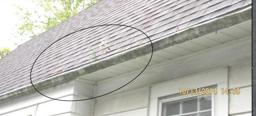
Obstructed gutters, more trash, the downspout empties at foundation and bent awning—all these issues hurt curb appeal.
