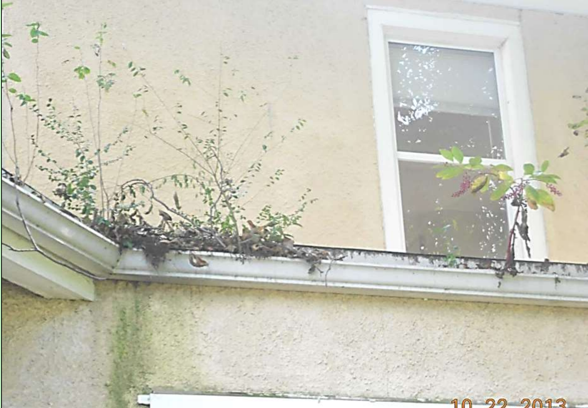
This gutter is severely obstructed with plants beginning to grow. Discoloration can be seen below the ineffective gutter.
