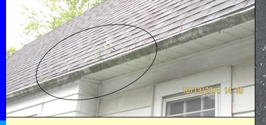
Obstructed gutters, more trash, the downspout empties at foundation and bent awning—all these issues hurt curb appeal.
