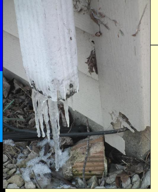
Fannie fails to replace the downspout diverter to protect the foundation from water damage or to replace the clip to keep the downspout in place.
