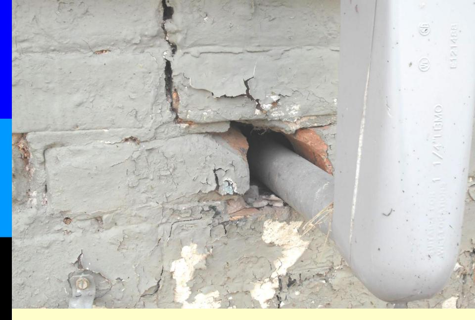
This hole in the foundation allows insects and rats or mice to enter the home.
