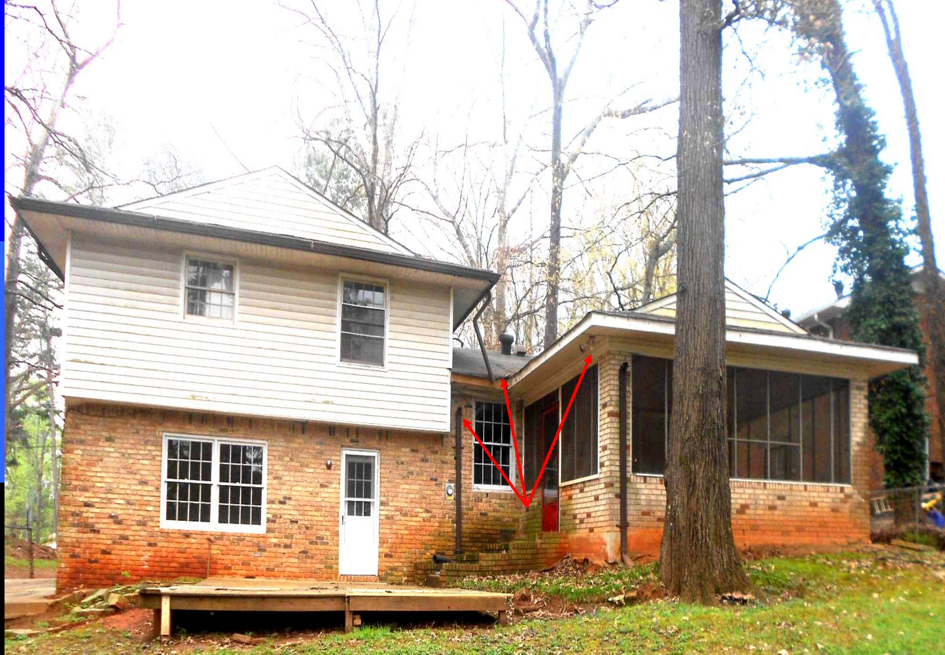
2015: Gutters and downspouts were missing or hanging all around the home.
